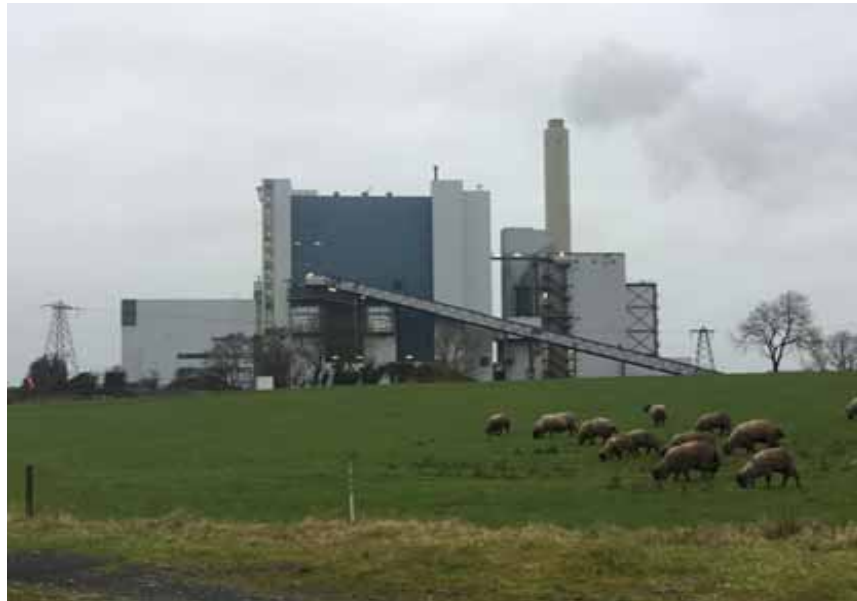
Lough Ree Power, Peat burning boiler, Steam Turbine, 100MW
