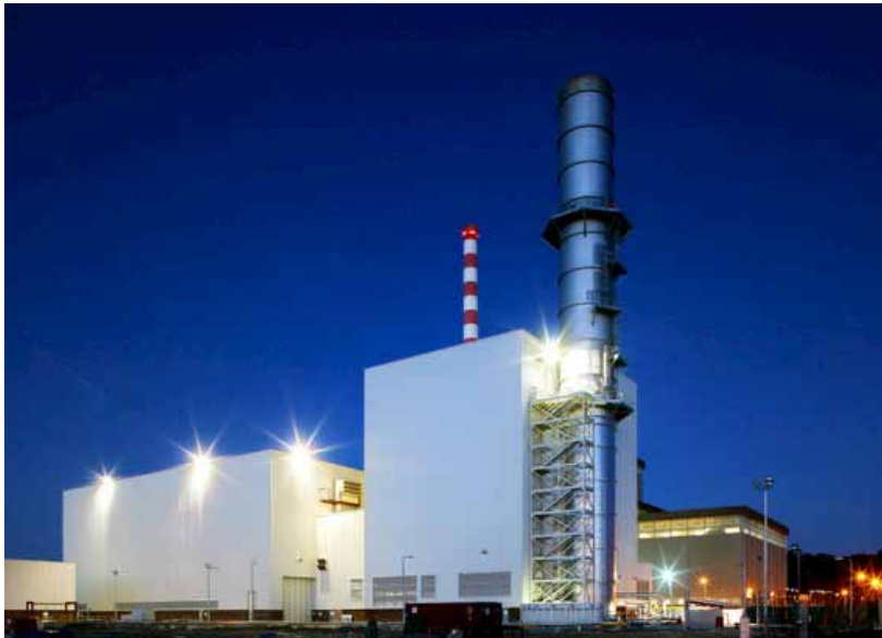
Aghada Unit 2, Single shaft CCGT 461 MW at generator terminals, 2010
